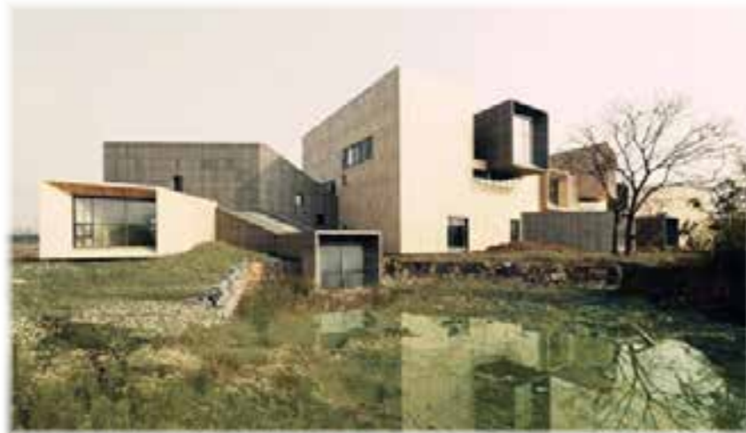
Typological precedent study #1 Xixi wetland art village / Wang weijen architecture (1.Projecting linear form / 2. "U" shape main circulation / 3. Reinforced concrete frame construction / 4. Function: various viewing frame / 5. Relationship of linear building massing)
