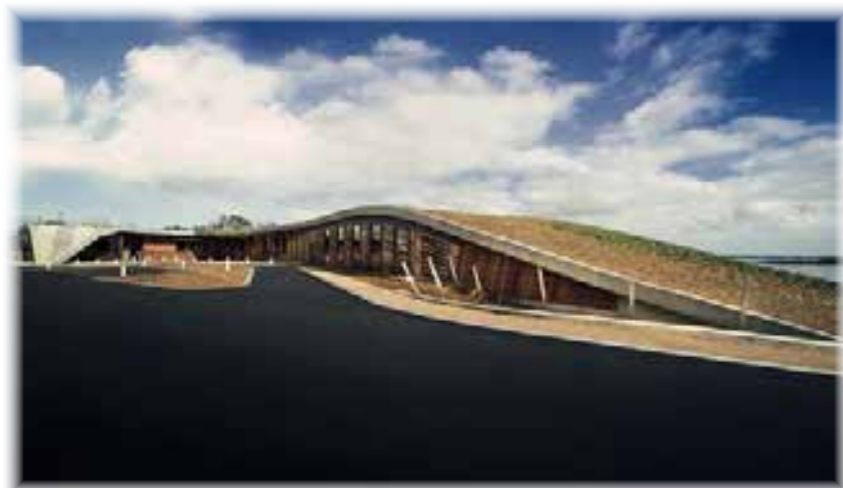
Typological precedent study #2 Marine and fresh water resource institute / Lyons architects (1.Linear form for fitting to the narrow site / 2. Concrete & steel structure / 3. Special construction for sustainable design (inclined wall as sunlight controller) / 4. Main circulation in main building block / 5. Relationship of rectangular building massing)
