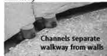
Water flows into channels that surround the elevated walkway
