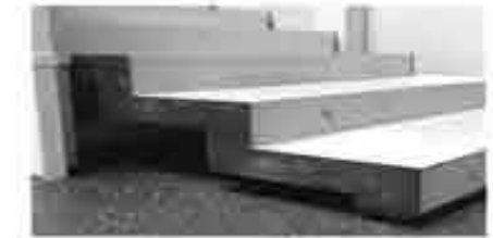
Hollow spaces below stairs allow flood going through
