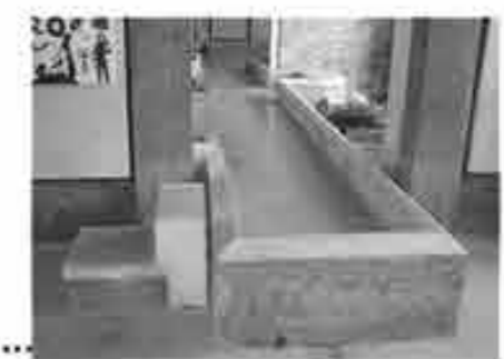
Water from canal is allowed to pass under the water gates into recess where a cascade of steps rise up to an elevated walkway.
