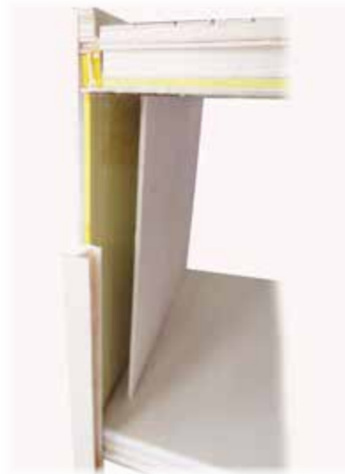
“Wall Construction: Mainly Shows Light-Weight Wall Construction And Load-Bearing Steel “H” Column.”
