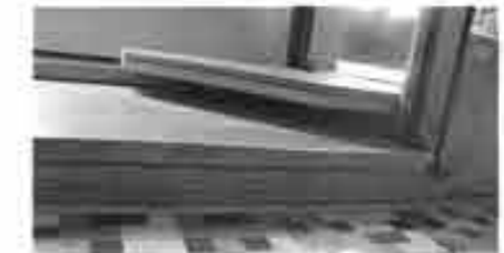
Hollow spaces below stairs allow flood going through
