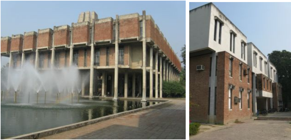
Figure 4: Library building showing structural framework and infill brick panels and skylight. (Source: Author 2011). Figure 5: Southern Lab complex (Source: Author 2011).
