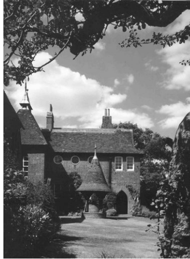
Figure 7. Phillip Webb's Red House, Bexleyheath, 1859-60 for William Morris. One of the works exhaustively studied by Spence. (Spence Estate, date unknown).
