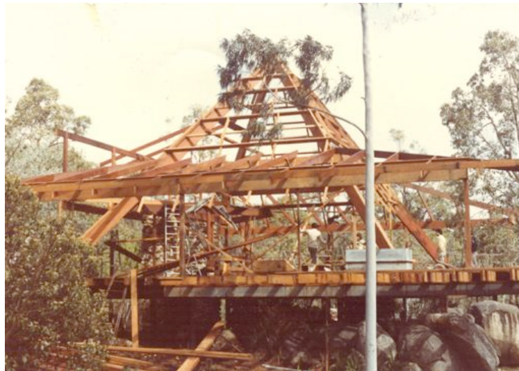
Figure 9. Pyramid House under construction 1984, Darlington. (Photographer N. Matthews.)
