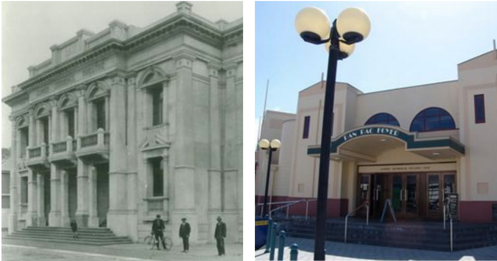
Figure 5. Entrance to the Municipal Theatre before 1931 earthquake.
