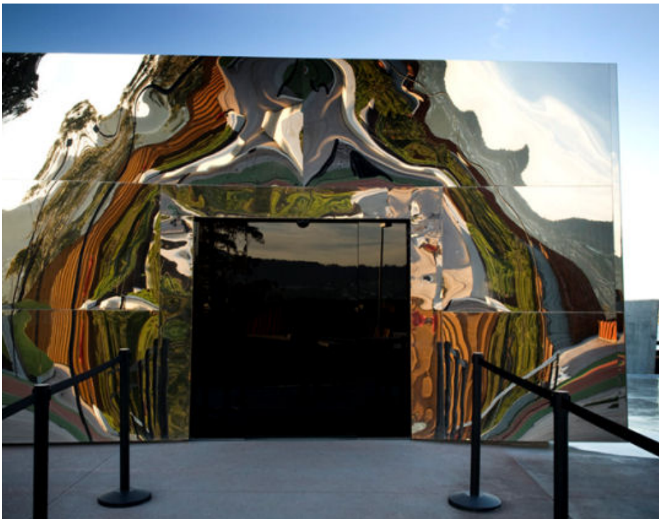
Mirrored wall on courtyard house, Photo credit: Matt Newton, Images Courtesy of MONA Museum of Old and New Art, Hobart, Tasmania, Australia
